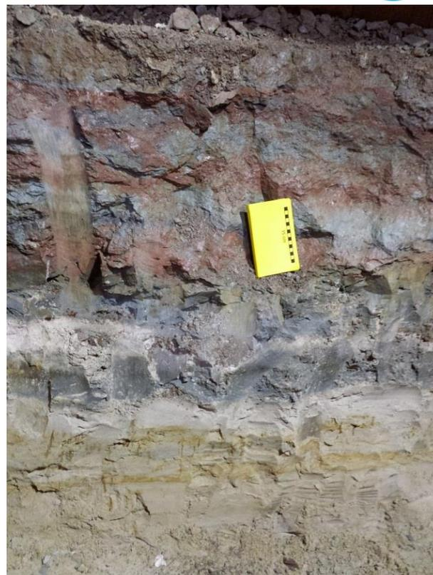
Photo 5. Dry non-cohesive soils encountered during excavation of CP6. (Left) Channel sands in the crown. (Right) Laminated beds at invert.
